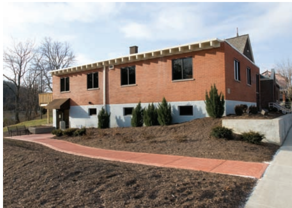
View showing newly excavated entry to Police Department
