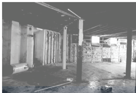
Before work began
