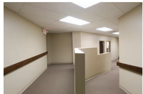
After completion—accessible and attractive
