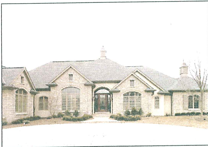
EGC designed and began building the 7,500-square-foot, Country French home on spec. The buyers entered the process in time to select most of the finishes and fixtures.
